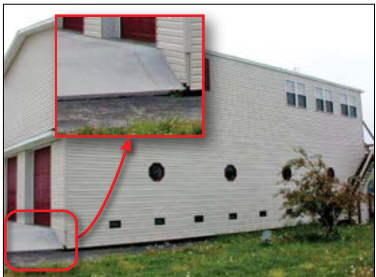
Figure 12: Manufactured home installed on columns above a full-height, framed garage (note elevation of thick driveway slab on left; the flood openings are within 1 foot of interior floor surface)
