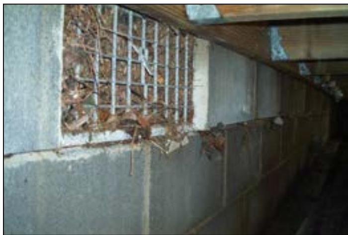
Figure 20: Typical air vents with insect screens blocked by flood debris
